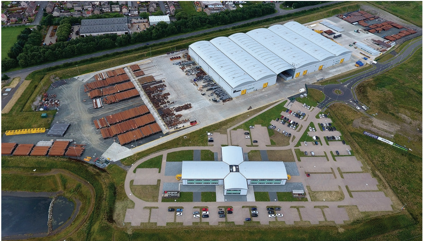
Oil States sales and manufacturing facility, Heartlands, UK.
