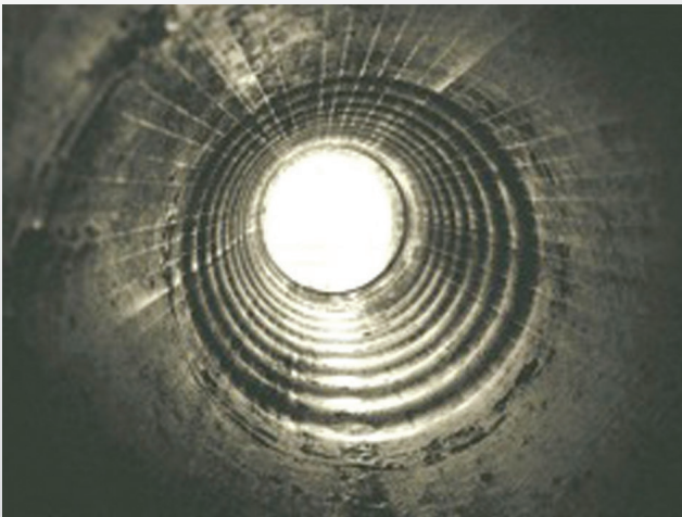
Internal view on completed Swage
