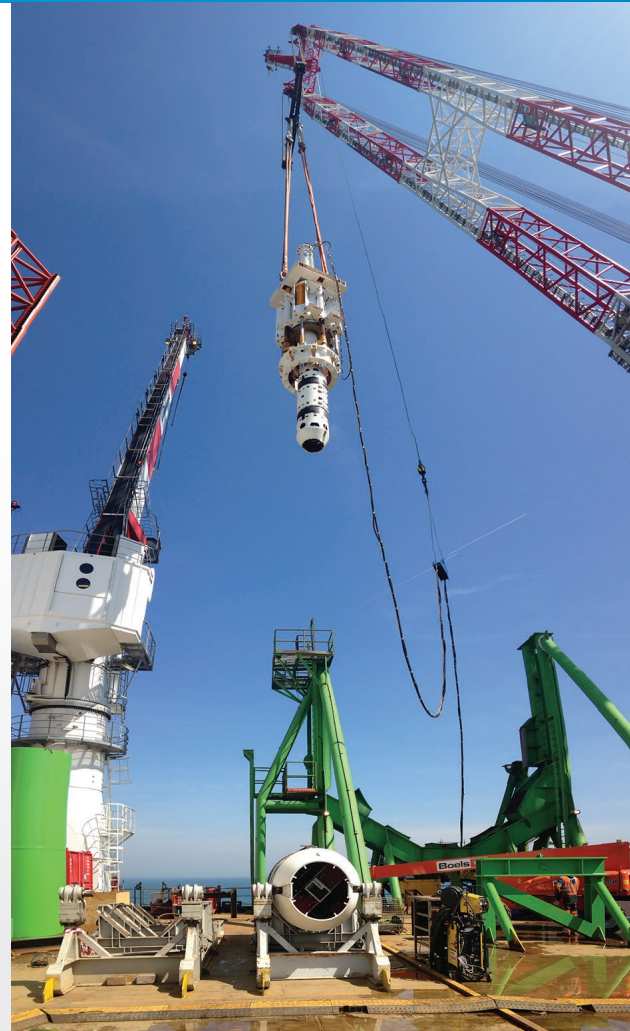
Single Operation Structural Levelling and Pile Connection using 60" HYDRA-LOK™ and Latch-Lok Jacking Tool
