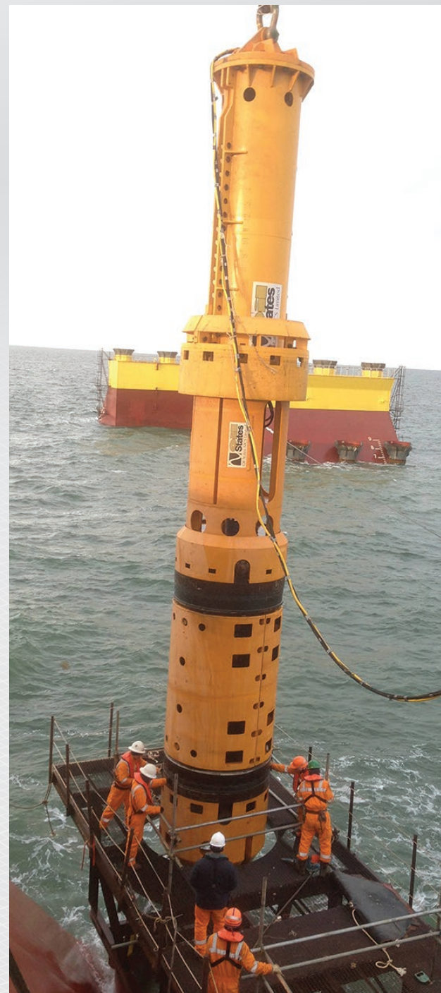
Ice Resistant Platform Installation – 84” pile connections
