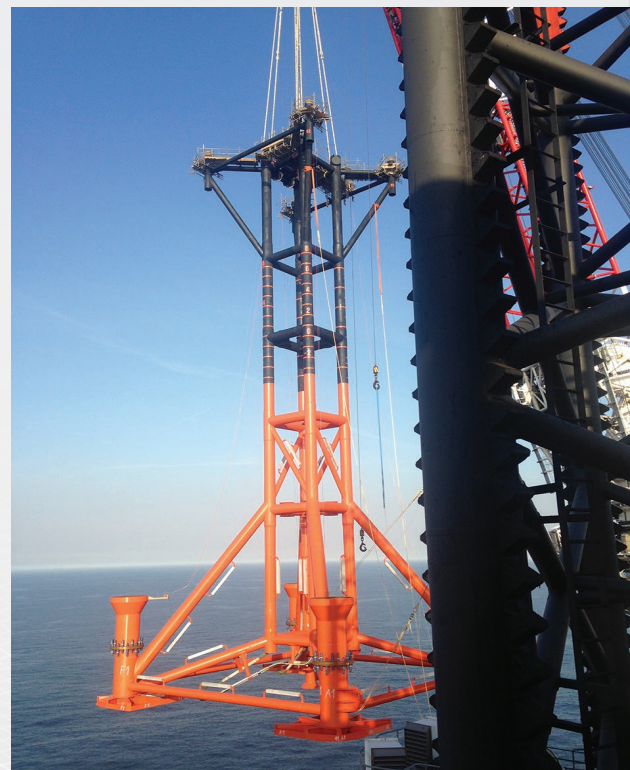
Jacket Installation in SNS 60" Swage Pile Connections
