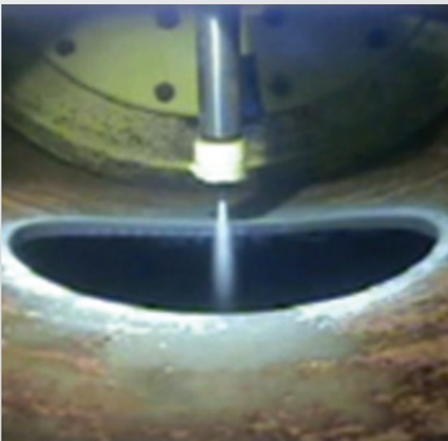
300mm diameter intake hole cut in caisson
