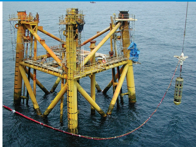
ICM Direct Deployment - Skirt Piles Cuts
