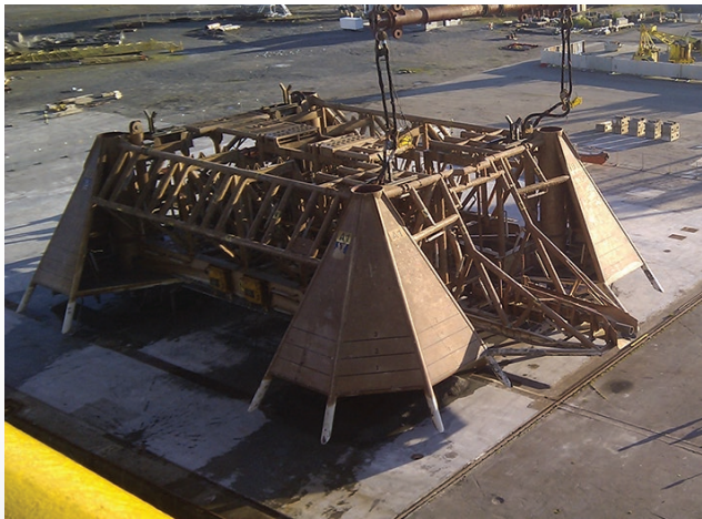
Togi Template Removal - 300m Water Depth Cutting
