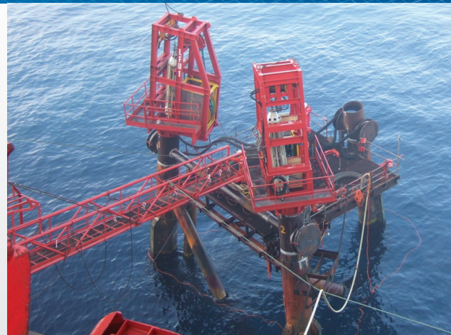
LFU deployed on tripod jacket
