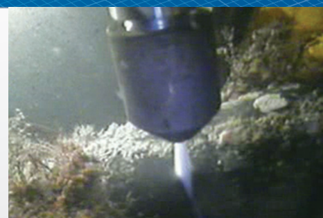
20" Pile cut & video monitoring of the Abrasive Water Jet
