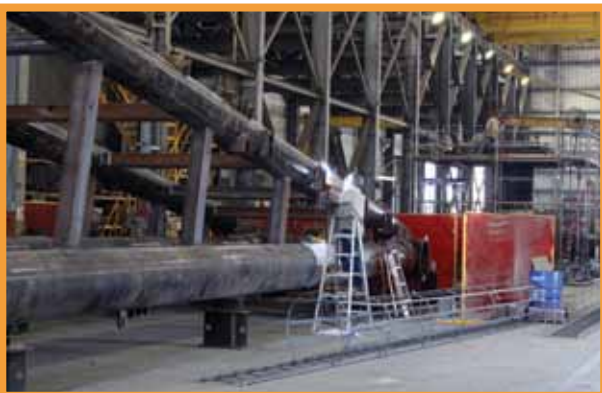
Custom Crane Gantry
