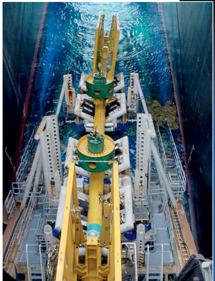
Mud mats being installed on a 16-inch x 20-inch Mid-Line Tie-In Sled for installation in a water depth of 5,100 feet .
