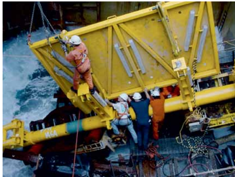
24-inch x 16-inch x 12-inch Inline Tee Sled with Mud Mats
