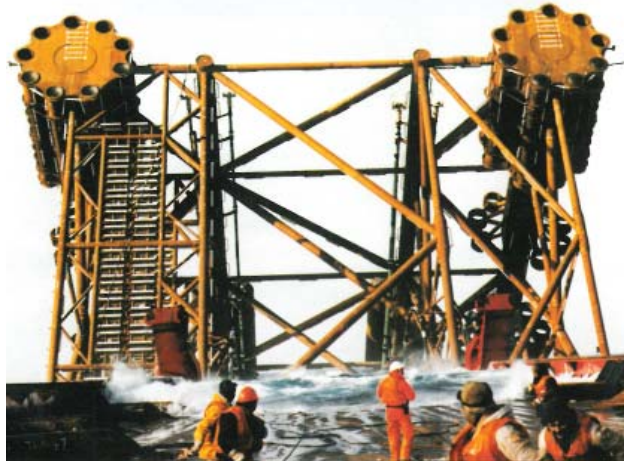
Photo courtesy Marathon Oil UK, Ltd. and Offshore Magazine Oil States' 87-inch diaphragm closures on Marathon's 21,000 ton South Brae A jacket.
