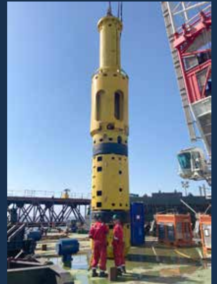
▲ ICE resistant platform installation - 72" pile connection
