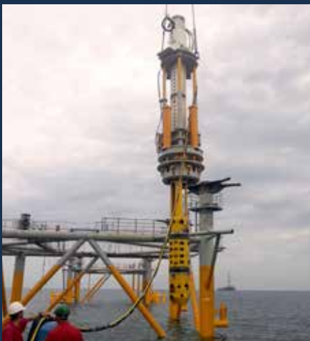
▲ 36" Levelling & swaging tool single deployment in the Dutch Sector North Sea
