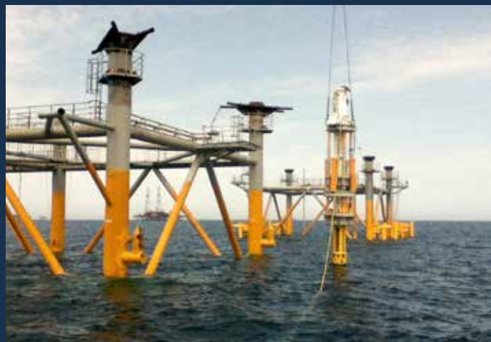
▲ 36" Levelling & swaging tool single deployment in the Dutch Sector North Sea
