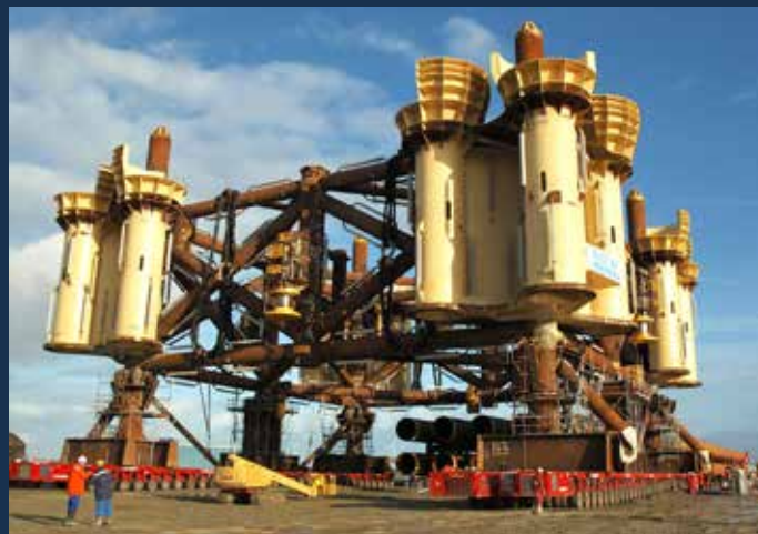
7,000 ton Jacket Template, levelled and swaged in Caspian Sea ▲
