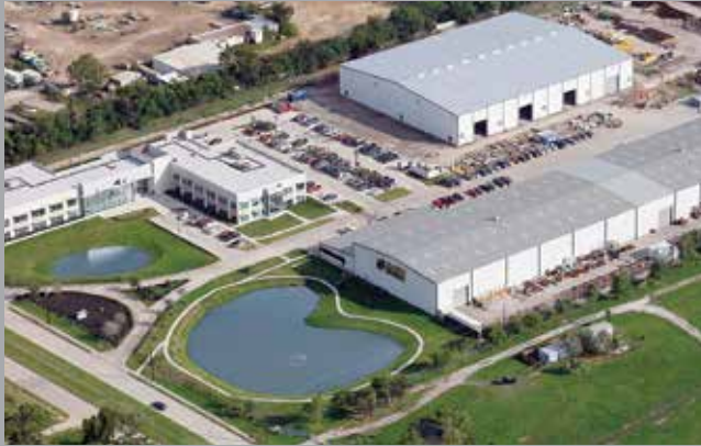
Oil States sales, manufacturing and service facility, Houston, Texas
