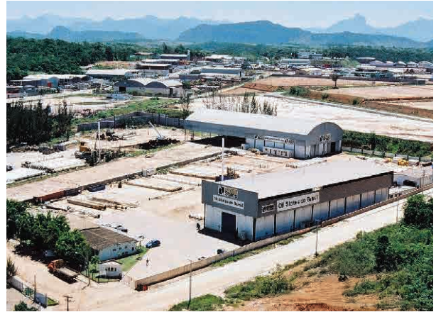
Oil States do Brazil - Cybersolda facility, Macaé, RJ Brazil
